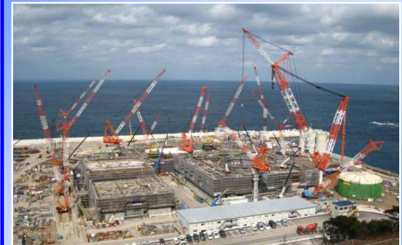
Shimane Unit No. 3 ABWR Construction Site Visit by Overseas Parties
