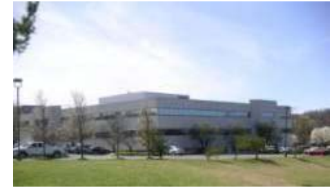
Hitachi Power Systems America [HPSA] (Established Feb. 2005)
